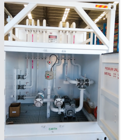
Pump bay with Unloading ULP / ULP98 pump
