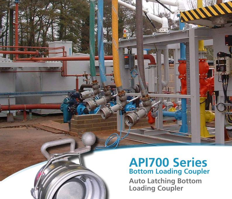
The API700 series of couplers is the third generation of Liquip manufactured API couplers, it provides an effortless automatic connection for a safe and environmentally friendly transfer of product from the loading rack to the truck.
